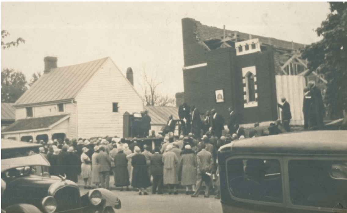
First Baptist Church during construction.
