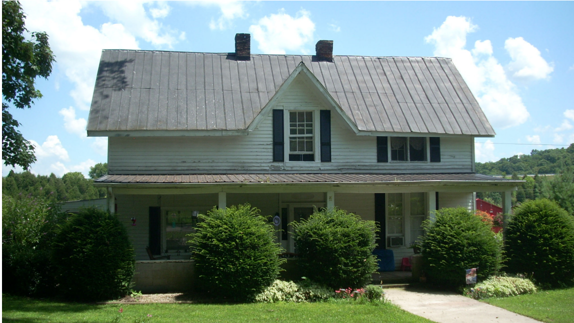
Surviving portion of the Blue Licks Hotel (Photo by the author)
